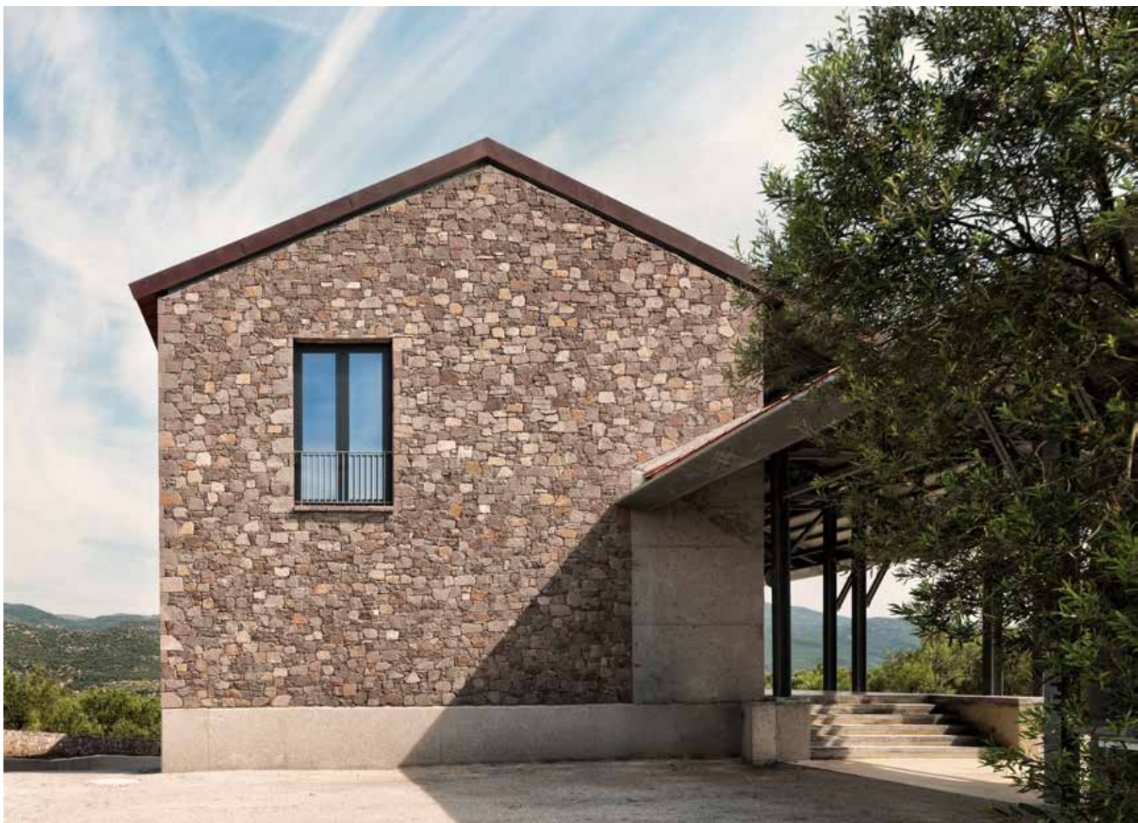
The main building and pressing area where olives are unloaded, weighed, and conveyed to production 橄榄的卸载、称重及榨油工序都在加工区完成。图为主建筑和加工区
